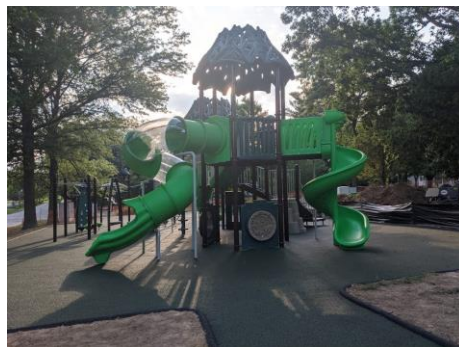
Photo after the safety surface was installed.
